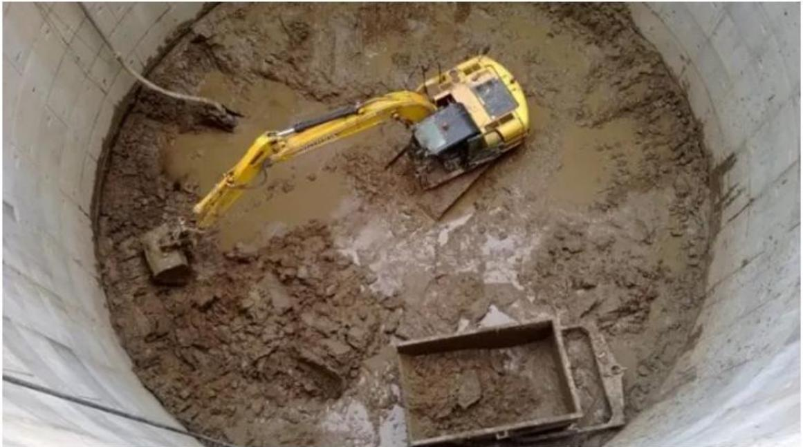
Figura I-2: Excavación mecánica de pozo vertical (<https://theconstructor.org/construction/excavations-groundwater-control-methods/17909>)
